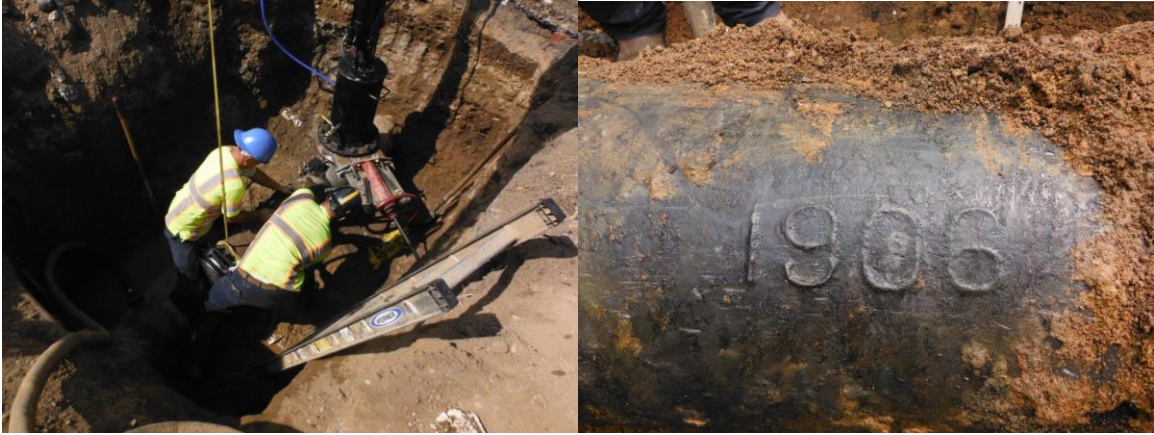
Line stop installation on the Square on some 100+ year old pipe.
