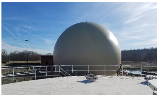
Digester Gas Holding Duosphere
