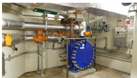
#1 Digester Heat Exchanger
