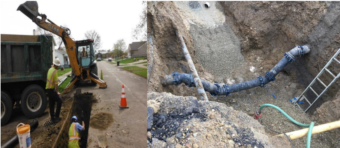
New 8" watermain on Arlington Ave. Horns Hill Rd. lowering for sewer.
