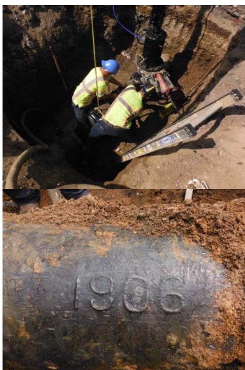
Line stop installation on the Square on some 100+ year old pipe
