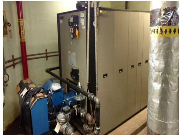
Boiler - Digester Heater
