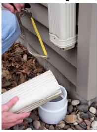
Step 1- Cut downspout from sewer pipe
