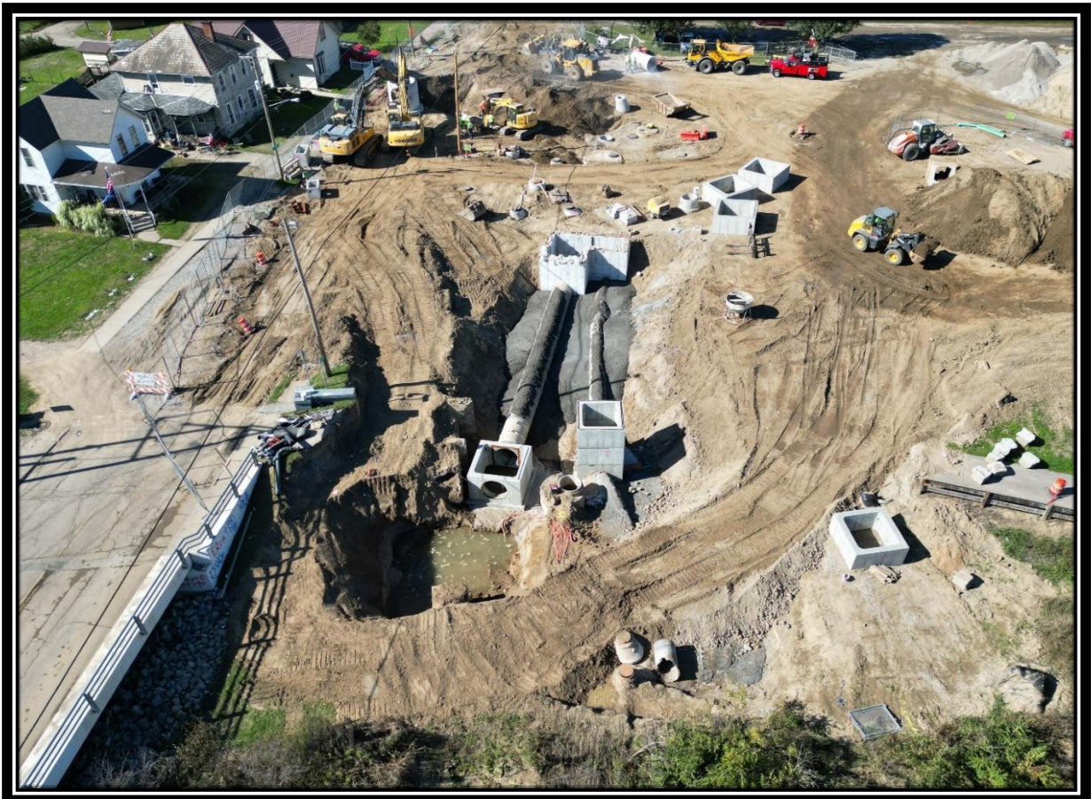
South 2 nd Street Sewer Separation Project
