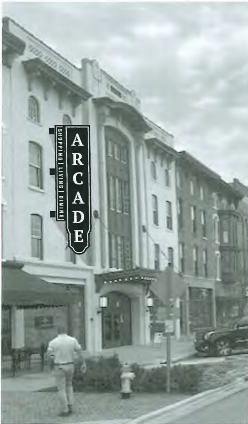
INDICATED ALUMINUM LED ILLUMINATED BLADE SIGN W/ PUSH-THRU ACRYLIC GRAPHICS ATTACHED TO EXISTING BUILDING
